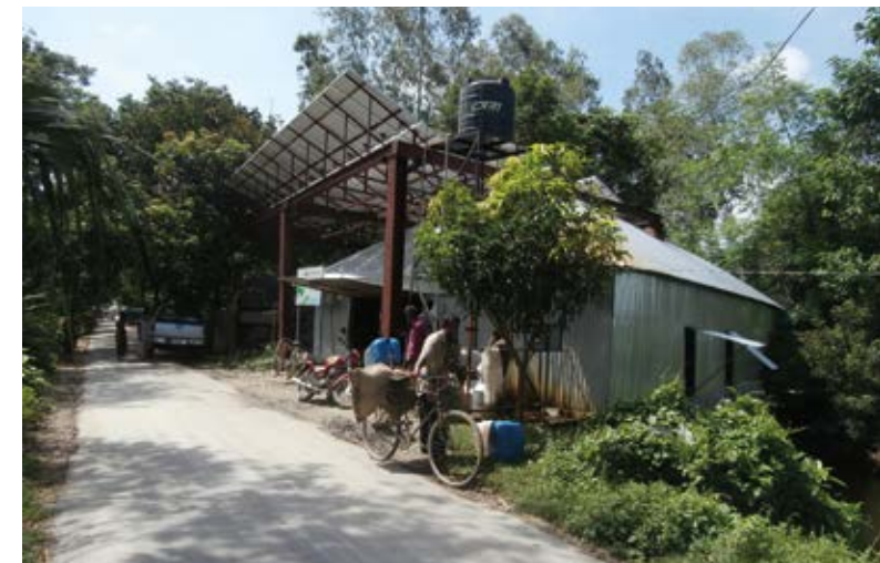
Left: An MCC in Goihatta, equipped with a solar installation and a solar water heater. Credit: Enerplus
