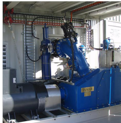
An example of a containerised mini-hydro; the technology that could be used for potential sites identified during the study.
